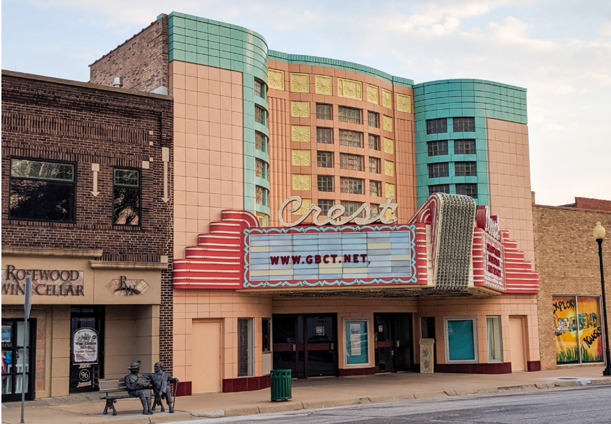
Our Great Bend crew worked with the Crest Theatre and neighboring businesses to conduct two separate night outages.
