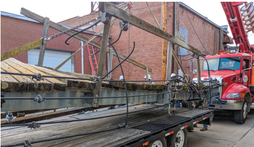
One of the old platforms that a transformer sat on is ready to be hauled away.
