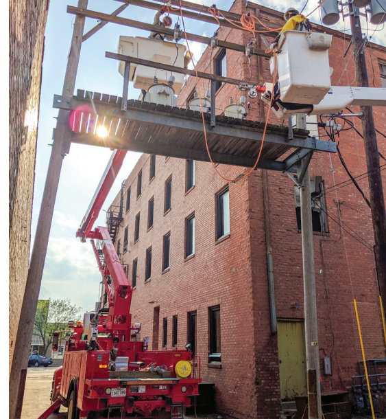
An older platform and transformers were removed from the alley behind the Crest Theatre in Great Bend during a night outage on May 30.
