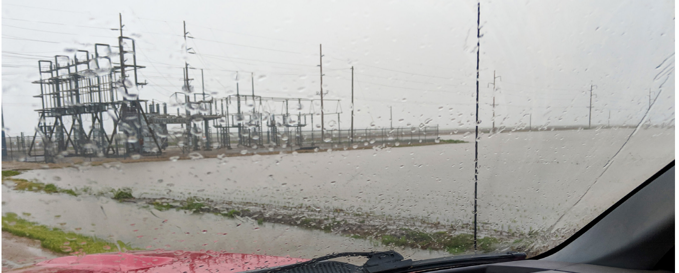
Great Bend crews look toward the Wheatland substation northwest of Great Bend after heavy rains fell in the area.
